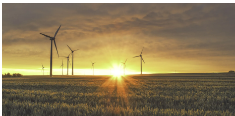
Wind energy avoided the emission of 28 million tonnes of CO2 in 2019.
